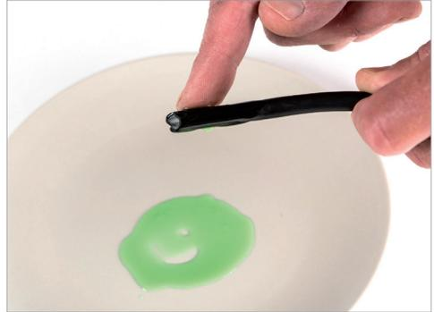
**1.2** Lubricate the cable cover with soft soap or similar product. This will ease up the process of getting the cable through the cable entry components. **Ensure that the cable is disconnected from eventual power sources.**
